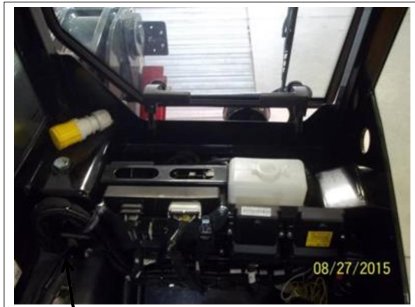
Hoses and electrical ready prior to cover and evap box being set in place
