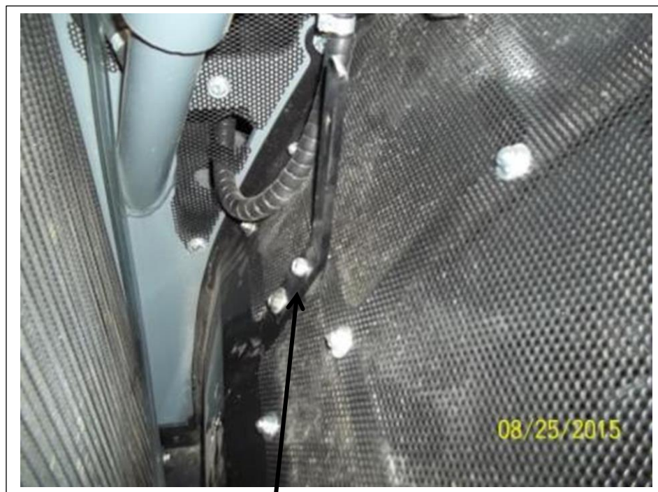
Drier bracket installed
