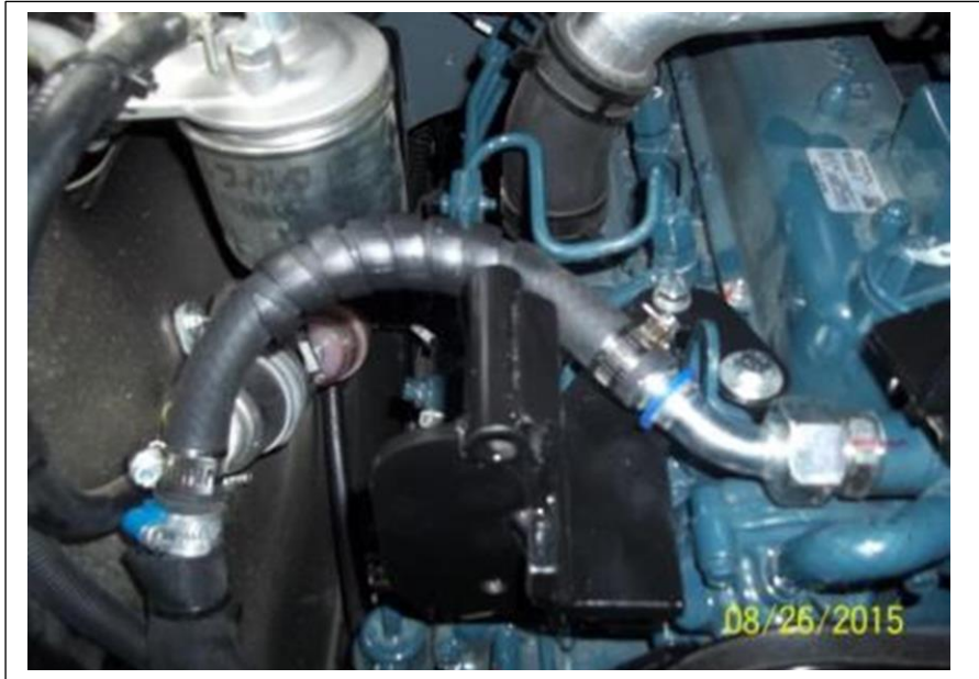
Heater hose reconnected after the compressor mount bracket was installed.
