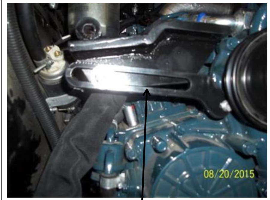
Compressor stiffener bracket installed.
